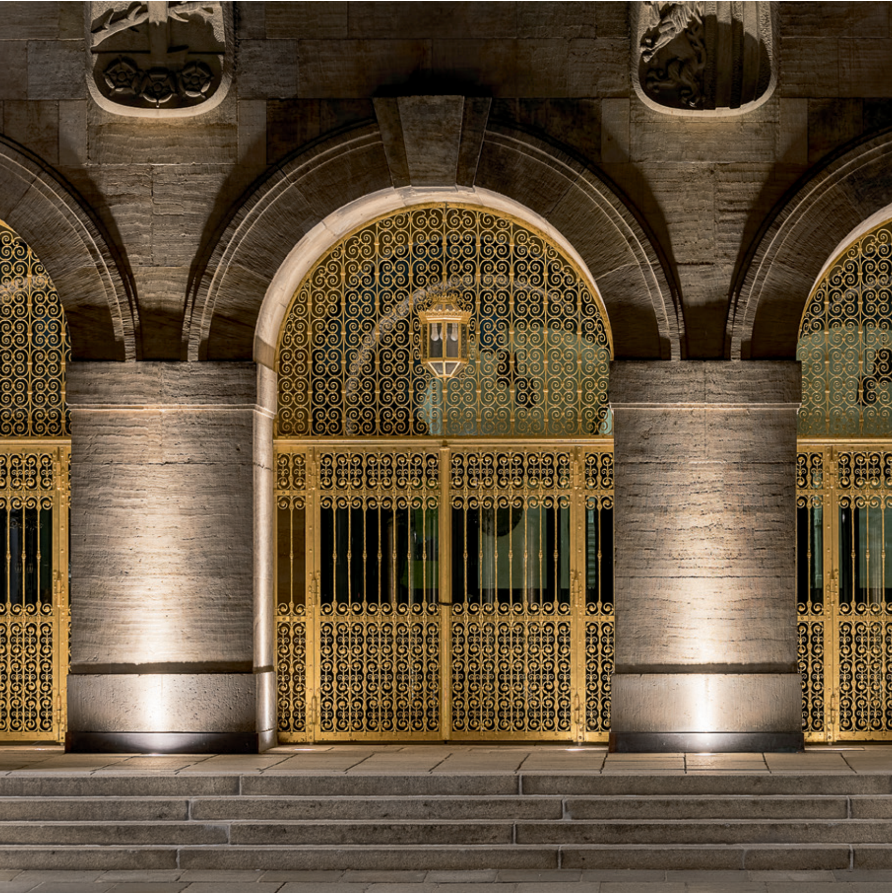
The Piece Hall. Halifax (UK). Architect: LDN Architects. Lighting design: Happold Lighting. Photo: Frieder Bickler. The shown application features uplights in close vicinity to a vertical structure, creating a 'column grazing' effect. Mood changes are achieved through 'smooth tuning' from 2700 K to 6000 K.
