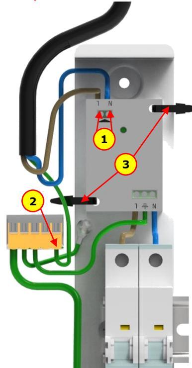
Connect Live and Neutral from luminaire to protected side of SPD (1), luminaire should be earthed to the tray (2), cable tie SPD onto tray (3).
