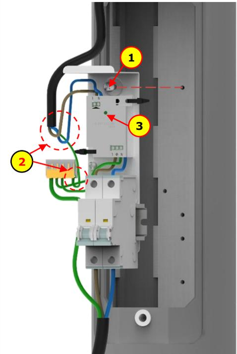
Secure SPD to pole tray using appropriate screw (1), luminaire cable should be **looped for anti drip (2)**. During operation, green light on SPD must be on, replace SPD if off (3).
