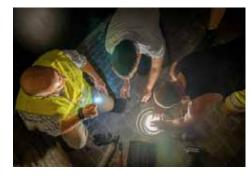
09 ETC130-GB and ETC140-GB are installed in the ground around the cathedral very close to the façade. Here, too, the WE-EF range offered the right lumen packages and light distributions for every lighting task.
