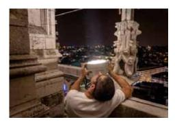
08 The projectors are used with different lumen packages and light distributions from wide to extremely narrow beam. In some cases, they are fitted with additional flood or wall wash lenses. Photo: © Fluvius Belgium (formerly Eandis)
