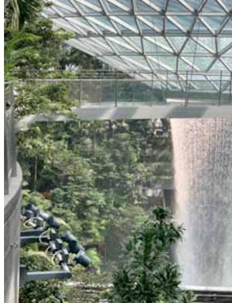
02 With viewing areas distributed over 360° and different height levels in the terraced park, particularly effective glare control was required. Almost all FLC projectors are equipped with glare shields.
