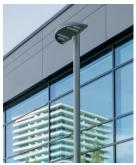
06 In the immediate vicinity of the façade, the poles are fitted with a semi-circular version of the RMC320 LED luminaire.
