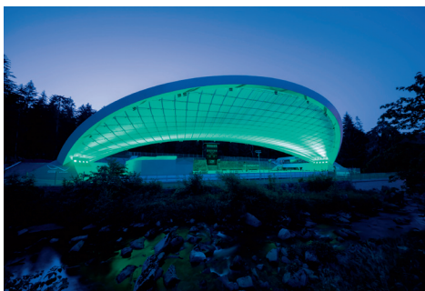
03 The structure, which rests on the ground at just two points, seems to float above the arena.
