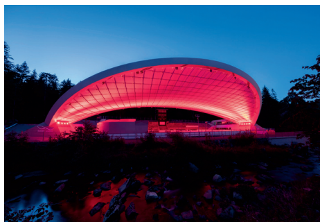
04 This impression is further enhanced by dynamic, coloured illumination of the roof on special occasions.
