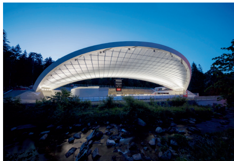
02 The extravagant, curved 2,400 m 2 roof comprises a steel ring structure spanned by a steel rope net covered with PTFE-coated glass fibre membrane.
