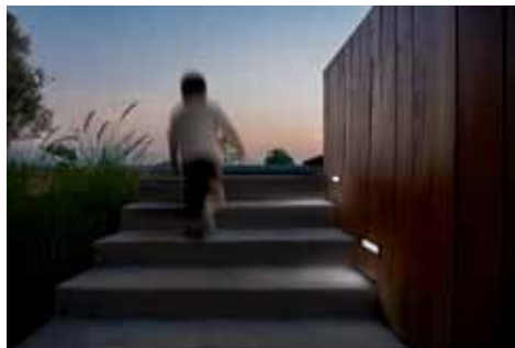
01 Recessed wall luminaires near ground level are important lighting tools for ensuring safe passage on dark stairs, ramps and terraces.
