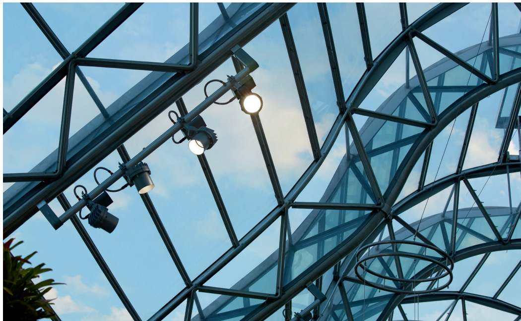
The Calyx, Royal Botanic Garden Sydney (AU) Architect: PTW Architects and McGregor Coxall Lighting design: Benjamin Cisterne
