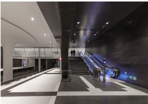
09 The planners adjusted the luminaire wattages and beam angles to the different ceiling heights of the hall and intermediate levels.
