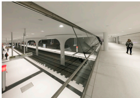
10 In the areas with lower ceiling heights there are more than 100 DOC220 recessed luminaires with 12 LEDs and symmetrical medium-beam optics.
