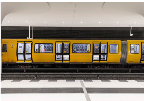
07 A total of 70 WE-EF type DOC240 luminaires with 24 LEDs in warm white (3000 K) and a connected wattage of a maximum 48 W are installed above the platforms.
