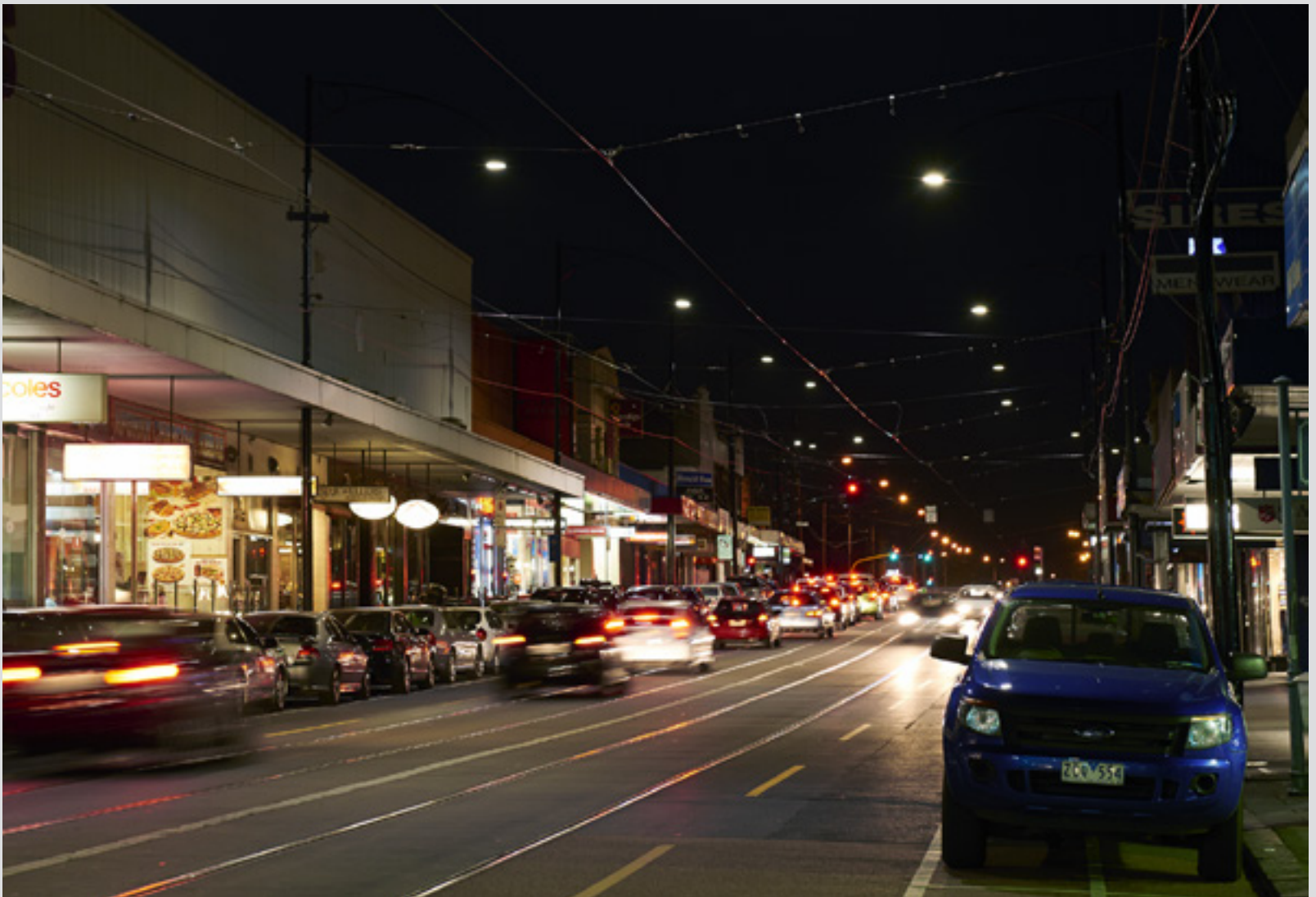
Sydney Road, Coburg, Victoria. V3 category lighting using ASP530 LED street and area luminaires.
