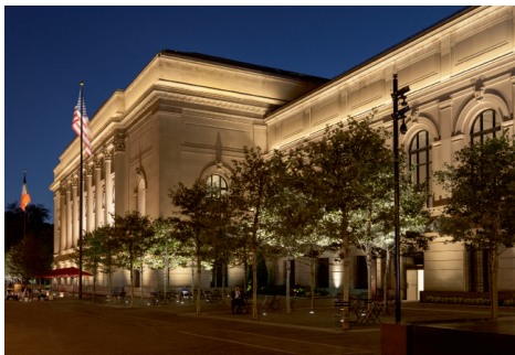
03 Metropolitan Museum of Art, New York, USA Architects (renovation): OLIN, Philadelphia Lighting Designer: L'Observatoire International, New York Photo: Alexis Nollet
