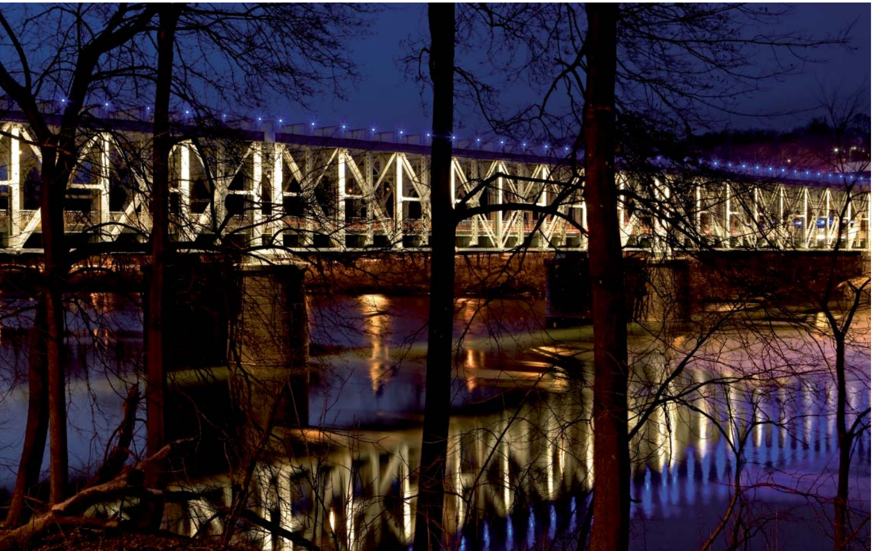
East Falls Bridge. Philadelphia (USA). Lighting design: Grenald Waldron Associates.
