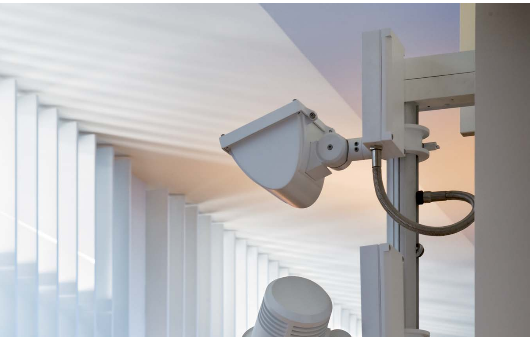
ASB Fitout. Auckland (NZ). Lighting design: Richard Bracebridge, Lightworks.
