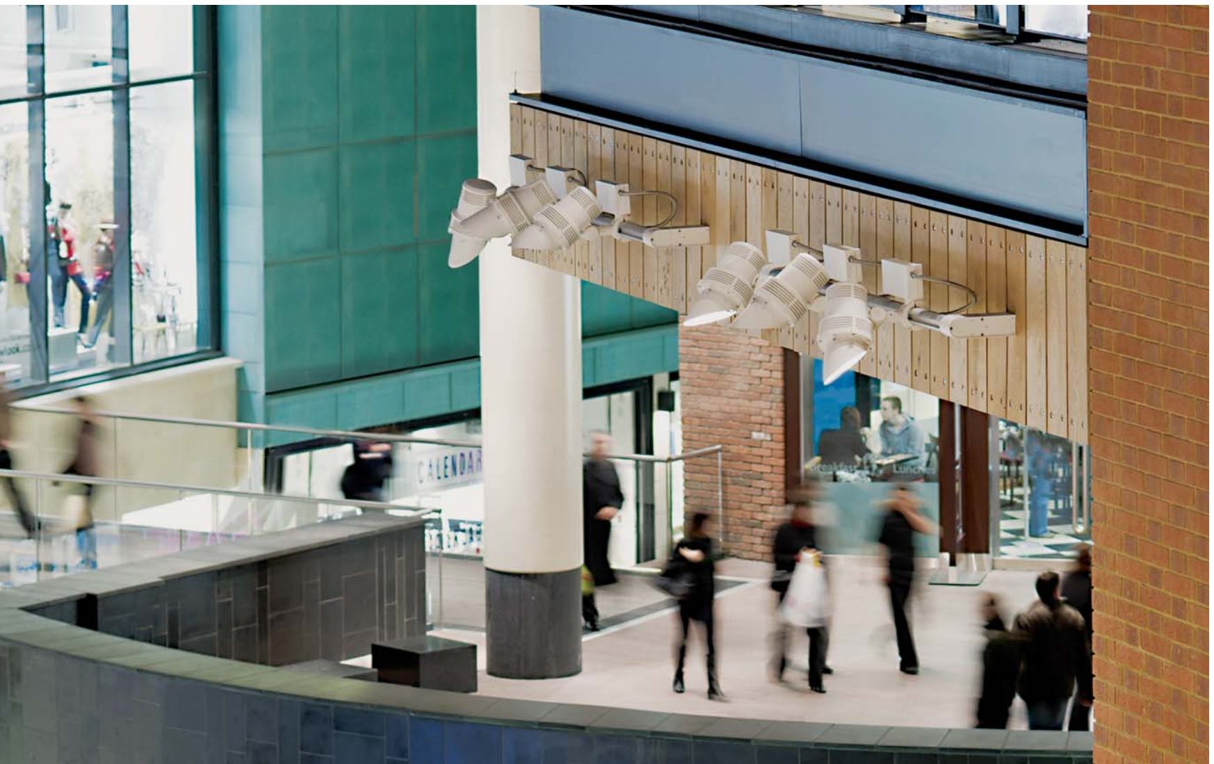
Cabot Circus. Bristol (UK). Architect: Chapman Taylor, Stanton Williams, Alex French. Lighting design: Pinniger and Partners.
