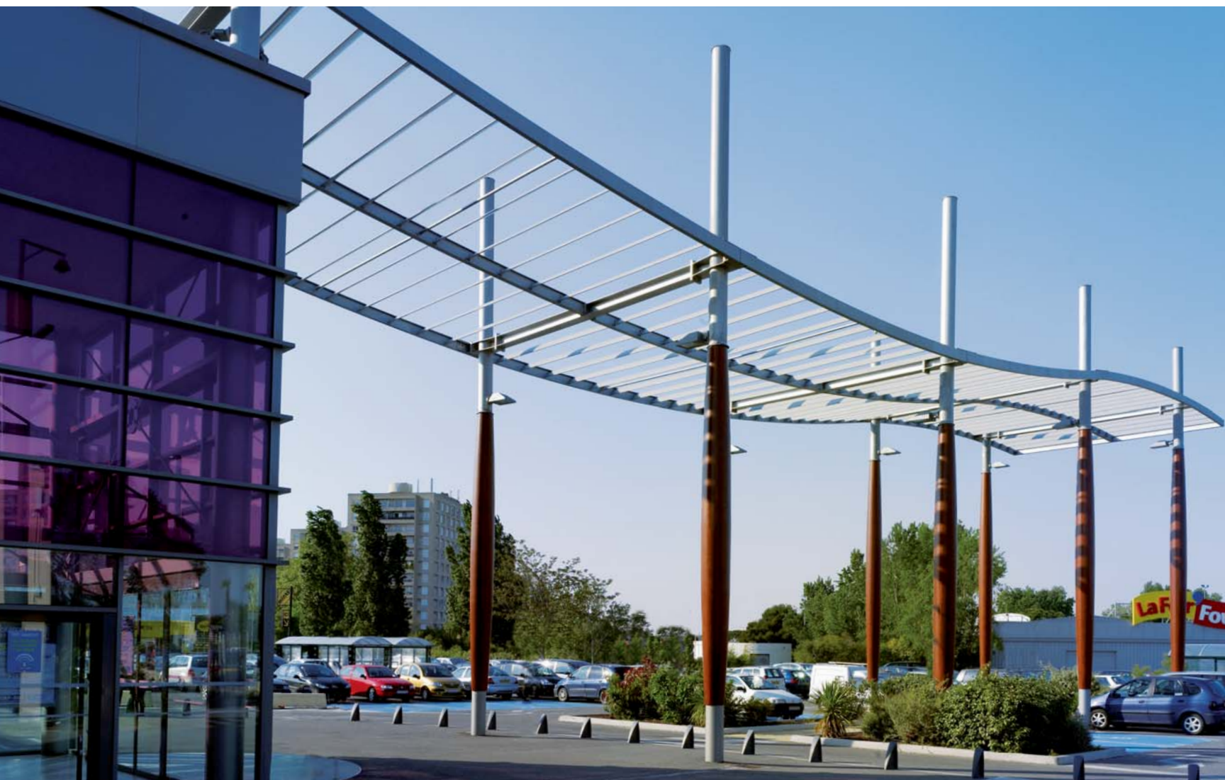
Shopping Center Cap Sud. Avignon (F). Lighting design: Acrobat, Saint Etienne.
