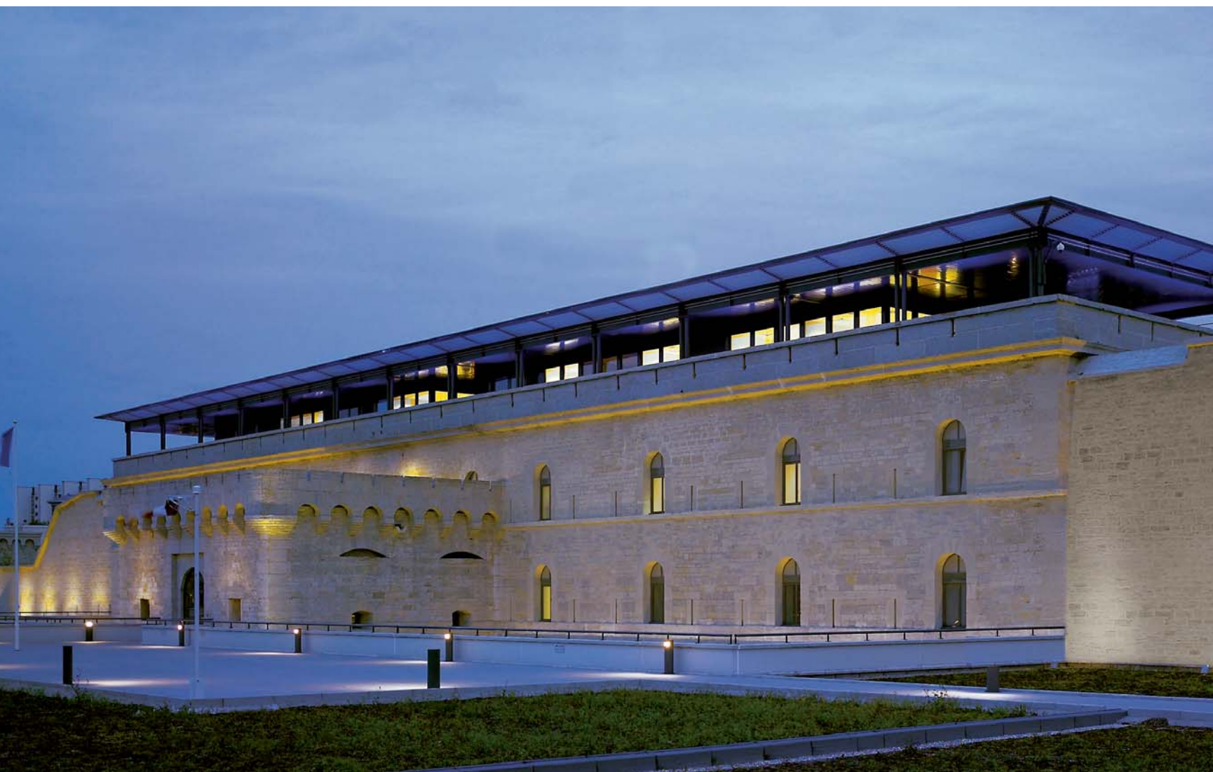
Fort Montluc. Lyon (F). Lighting design: Cobalt.
